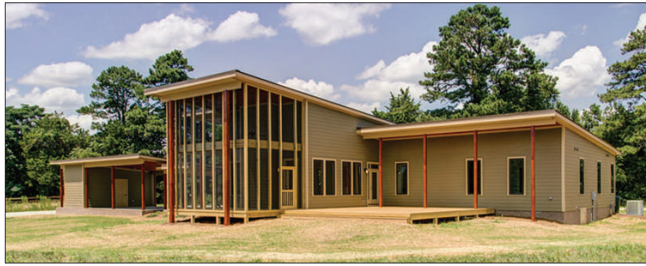
The home was sited in a pasture to blend with the natural environment and oriented to catch breezes and minimize windows facing west.
